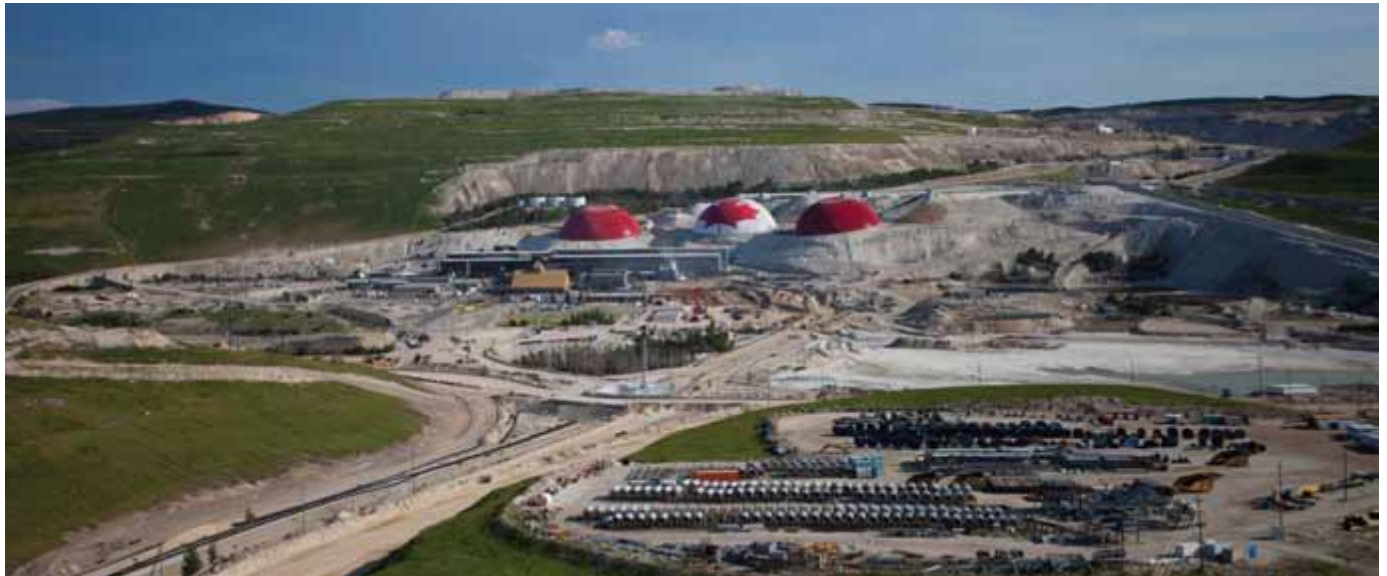
Highland Valley Copper Mine near Logan Lake, BC
