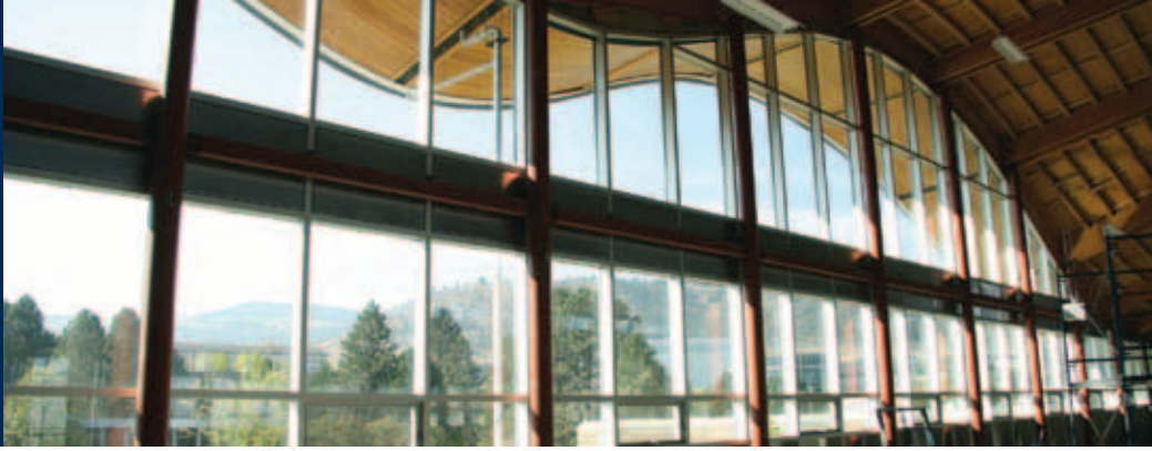
40,000 square feet of new learning space is under construction in Old Main
