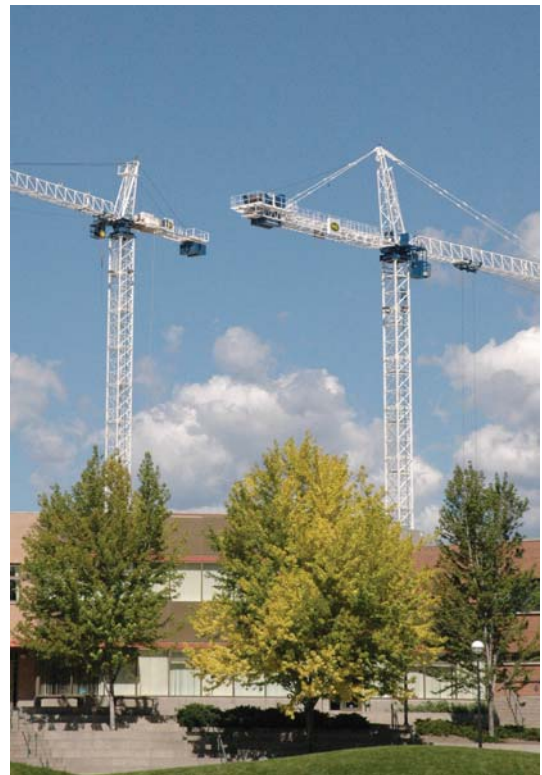
Cranes at work on the new residence building.
