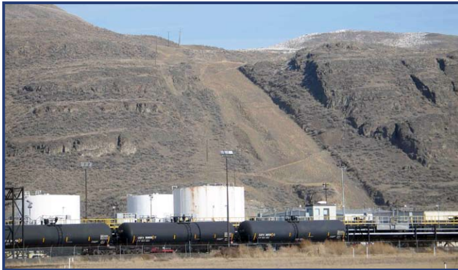
Figure 50. The smoothed and revegetated scar marks the buried route of the Trans Mountain Pipeline up the valley slope north of the petroleum depot and airport. The pipeline transports gasoline and diesel, each in separate batches, over 1000 kilometres from refineries in Edmonton via Kamloops to Vancouver and Washington State. The 60 cm diameter pipeline is owned by Kinder Morgan Ltd. and can transport over to 250,000 barrels of oil per day. (Photo by R.Turner)
