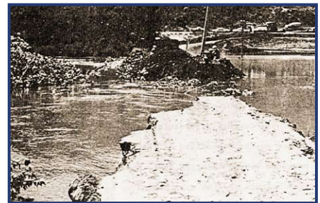
Figure 24b. Breached dyke at the Oak Hills subdivision during the flood of 1972. Photos courtesy of R. Buchanan and B. Gerath.
