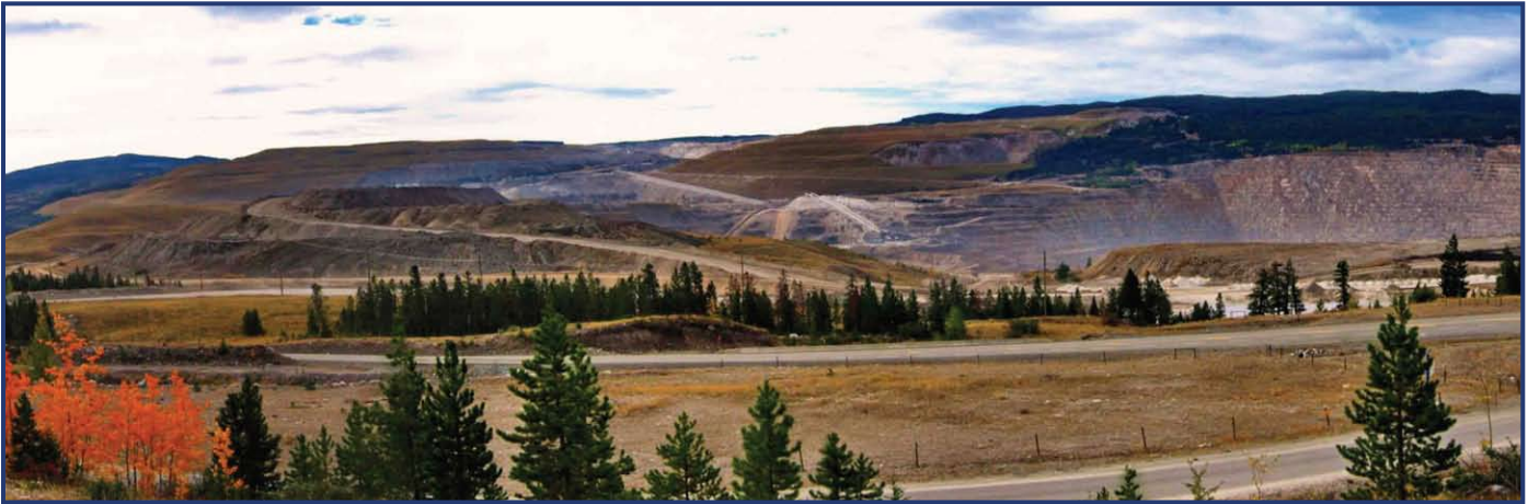
Figure 36. The view looking south of the Highland Valley open pit copper mines from the visitor viewpoint along Highway 97C west of Logan Lake. From right to left, the following features are in the far distance of the photo: the terraced rock wall at the top of the Valley mine pit; the white line of the conveyor belt that moves crushed rock from the pit to the mill; and golden grass slopes that cover reclaimed waste rock dumps upslope of the conveyor. Active waste rock dumps are in the middle distance, to the left of the conveyor. (Photo by R. Anderson)
