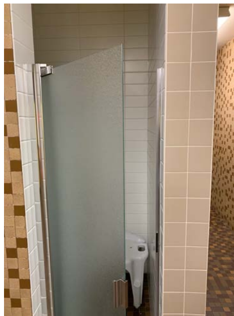
Photo 6.3-2 Frosted Shower Door in Gym
