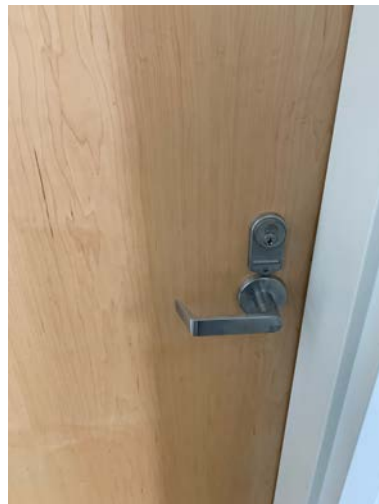
Photo 6.2-4 Lock without Occupancy Indicator in Industrial Training
