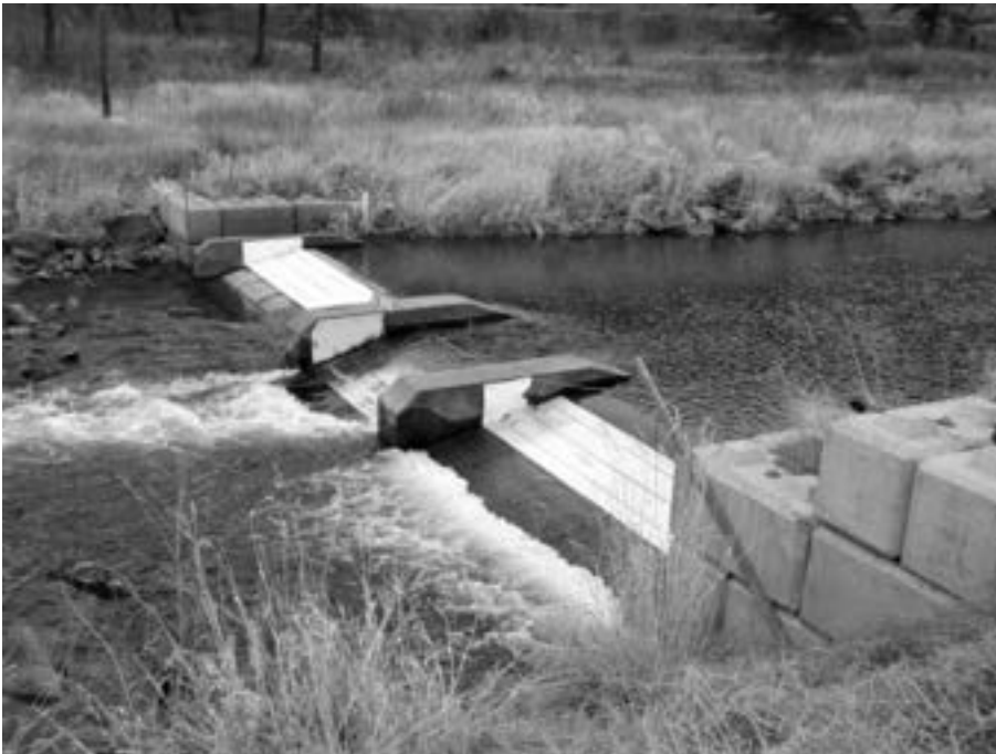
Figure 2-1 Deadman River resistivity counter at low flow (photo by author)
