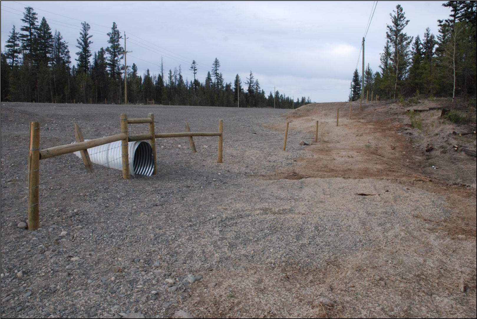
Figure 3.1. Recently installed badger-specific underpass crossing structure along Highway 97 south of 100 Mile House BC, Canada, 2010.
