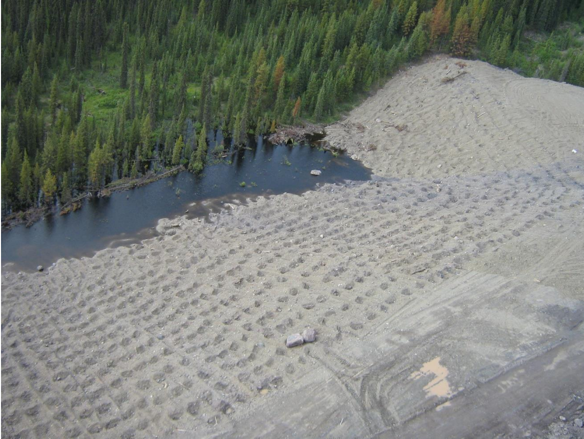
Figure 2.4: Study located on mounded waste rock storage facility at AuRico Metals' Kemess Mine site.
