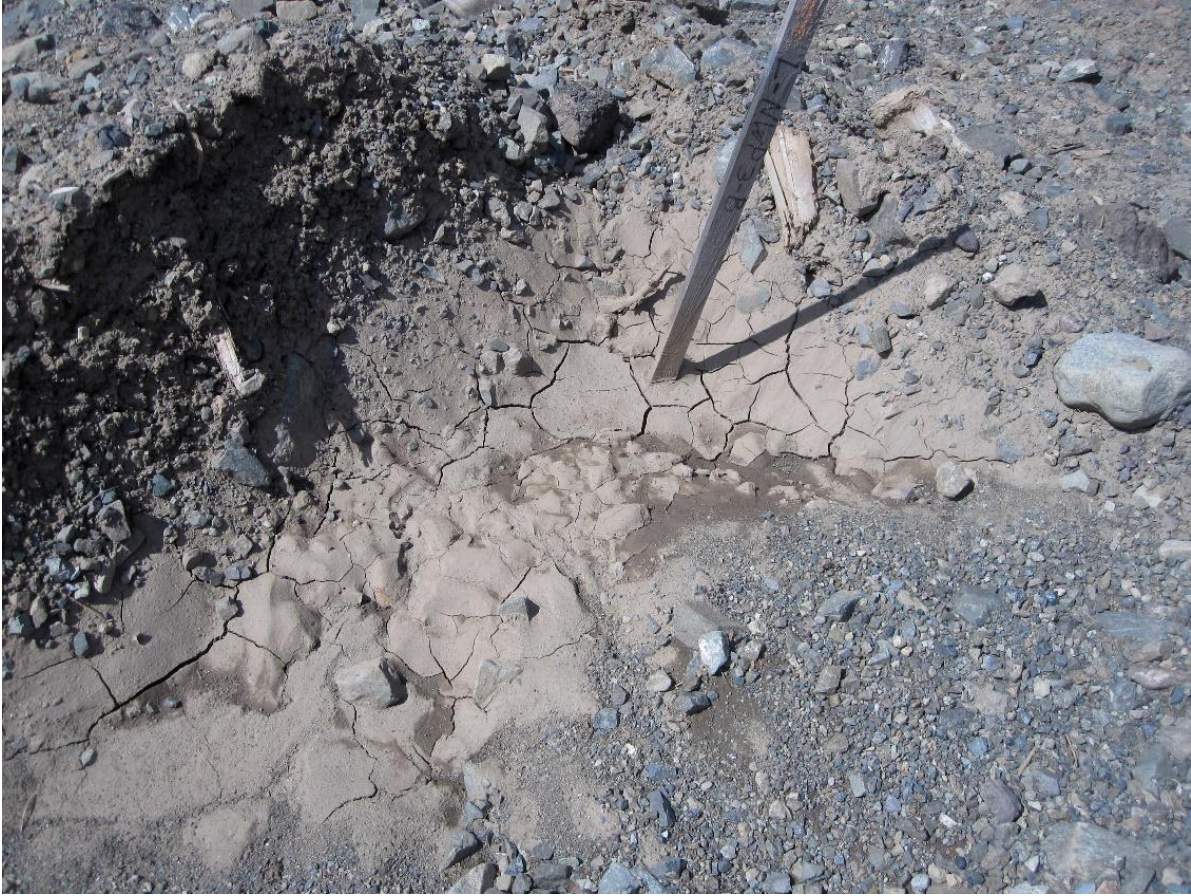
Figure 2.7: Bottom swale after standing water seeped into overburden.
