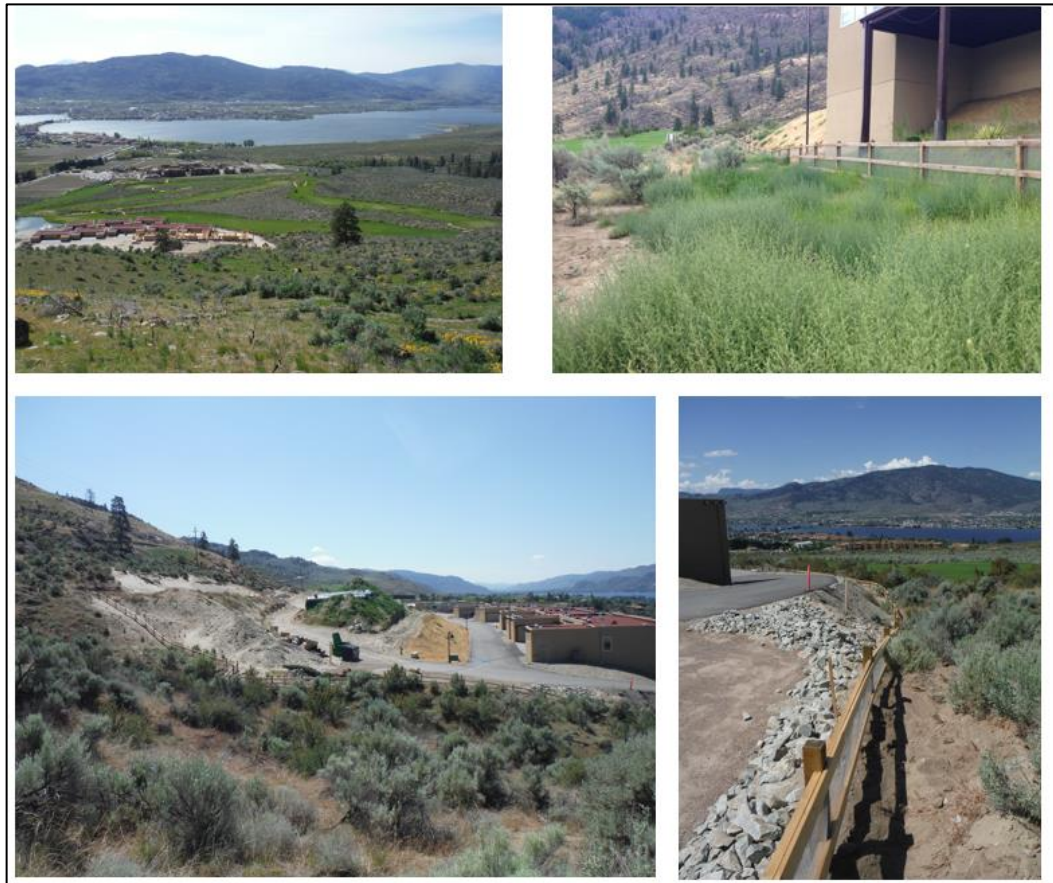
Figure 1.8. Condominium community and construction surrounded by a wooden, permanent snake exclusion fence.
