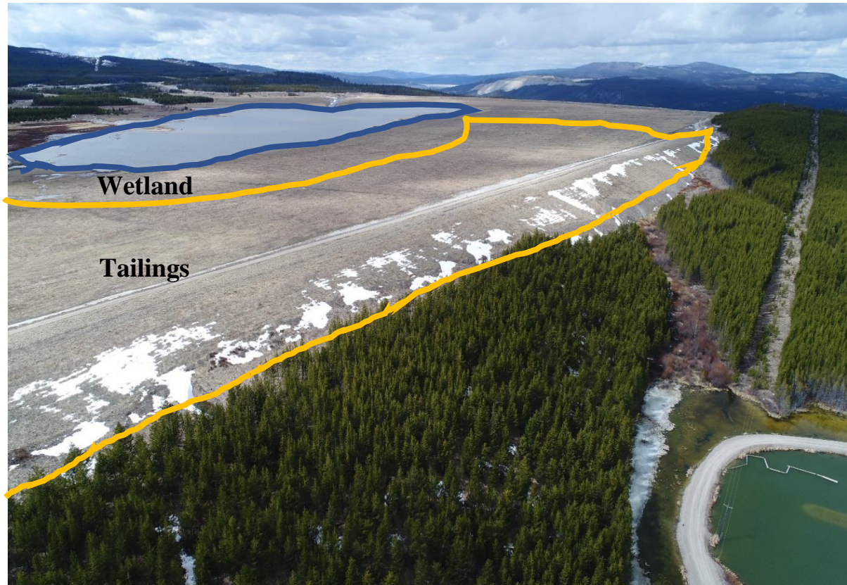
Figure 1.3. Overview image of the closed tailings facility (Highmont Tailings) located at Highland Valley Copper Mine located in British Columbia, Canada
