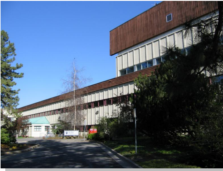
Old Main Building Before Renovation
