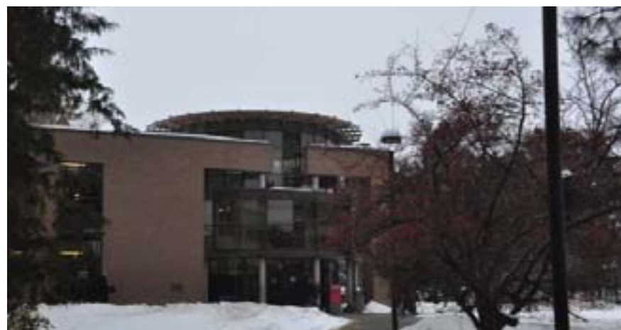
Main Library (built 1975)
